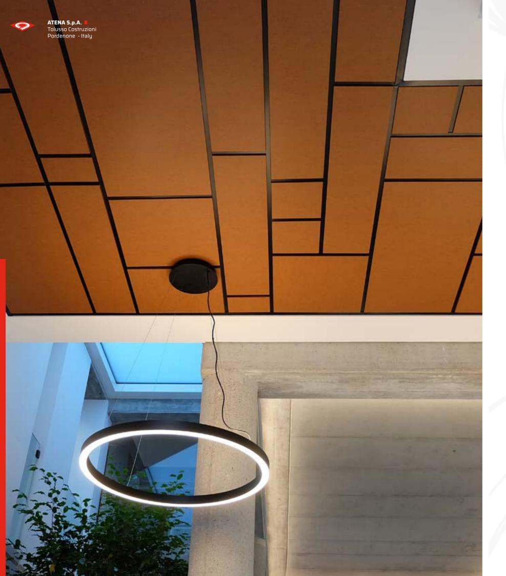
The particular arrangement of the metal ceiling, using **Atena Multipitch profiles**, was chosen for the **office** and **conference areas**, resulting in modular suspended ceilings with **panels of various sizes**.
