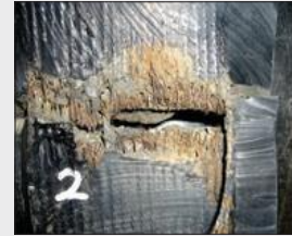
Steel cord breakage caused by rust
