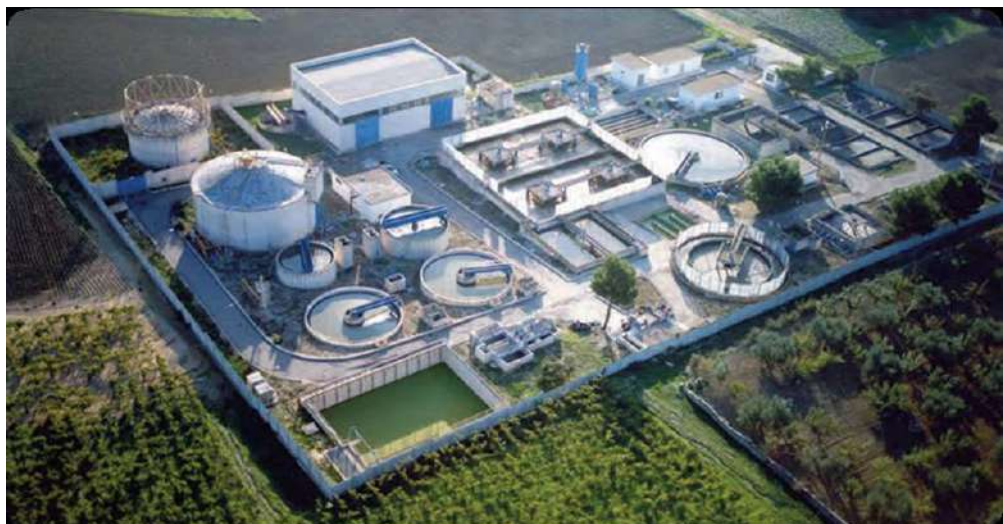
Mottola (Taranto) wastewater treatment plant
