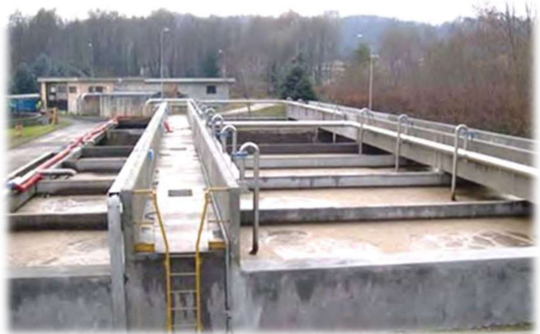
Borgomanero (Novara) wastewater treatment plant
