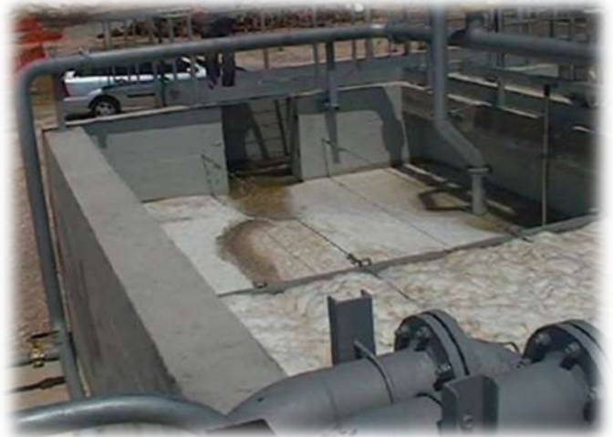
Works for a first functional lot are concluded.
