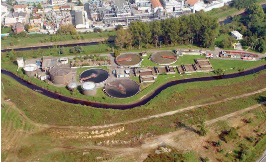
Rozzano (Milan) wastewater treatment plant
