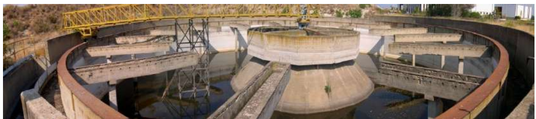
Megara (Syracuse) potabilisation plant
