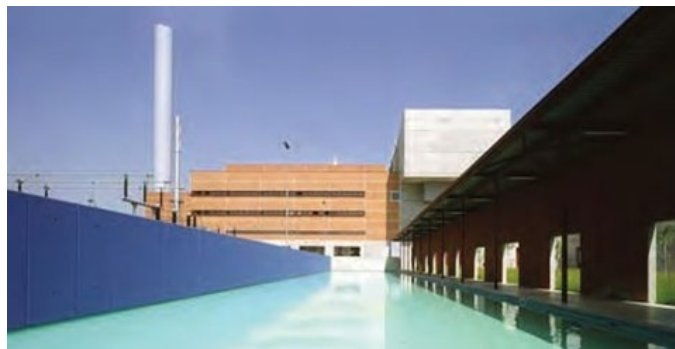
Silla 2 (Milan) waste to energy plant
