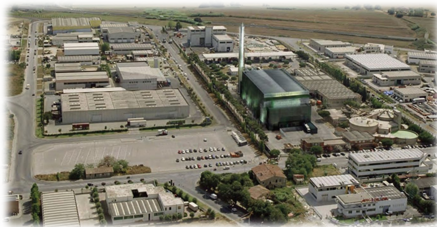
Leghorn waste to energy plant
