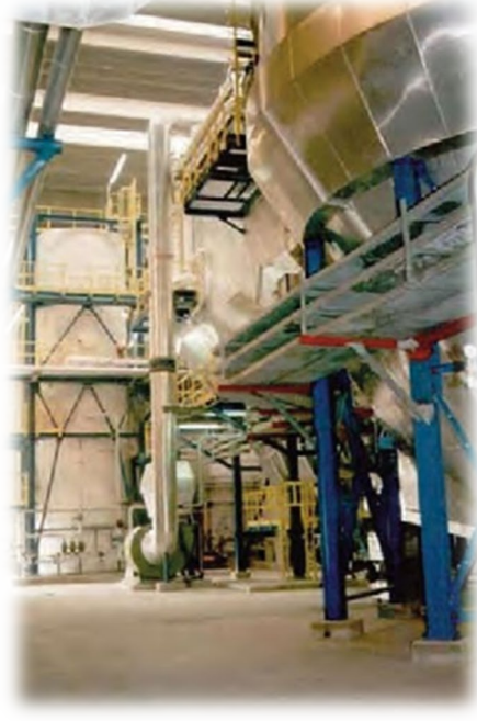
Busto Arsizio waste to energy plant
