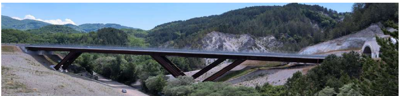
Viaduct Pineta - L= 175 m
