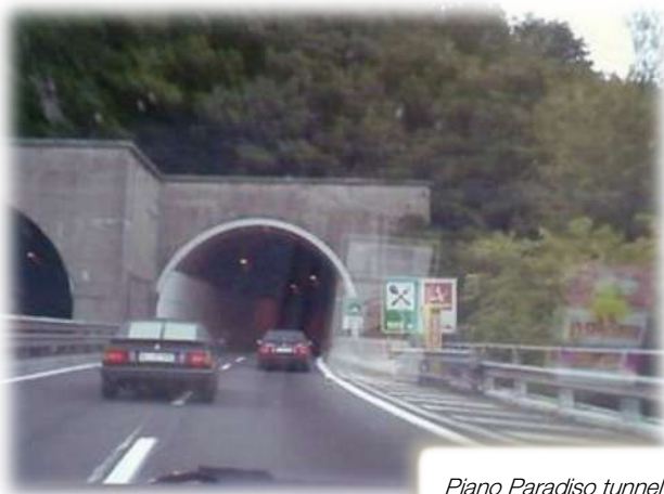
Piano Paradiso tunnel
