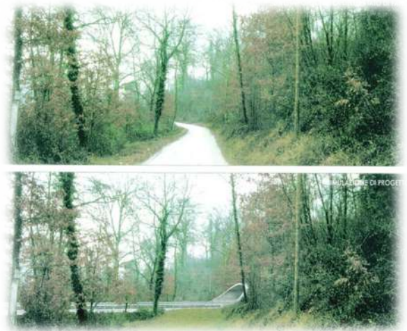
Tunnel entrance before and after the works
