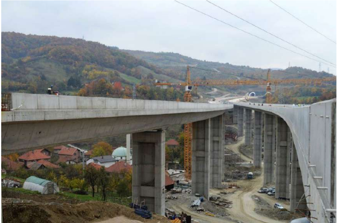
Double carriageways viaducts – Bosnia and Herzegovina
