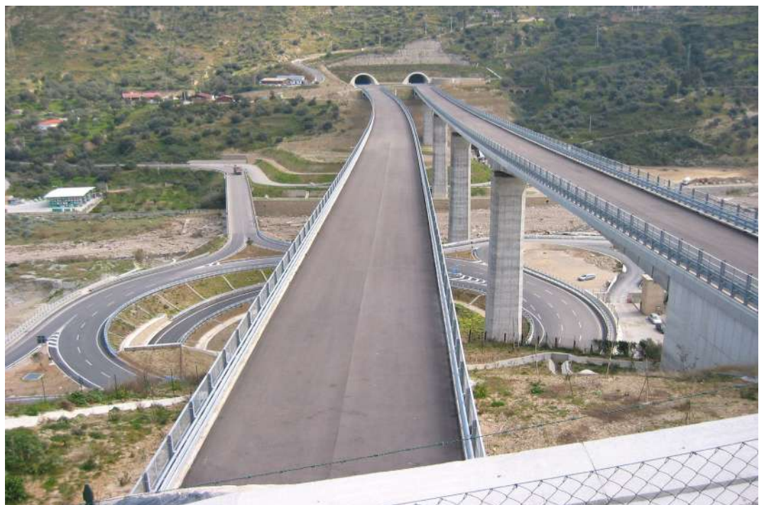
Messina-Palermo Motorway – Italy
