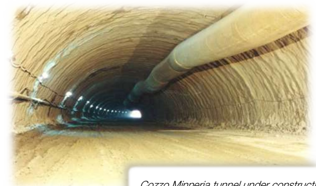
Cozzo Minneria tunnel under construction
