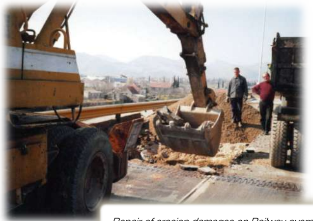
Repair of erosion damages on Railway overpass
