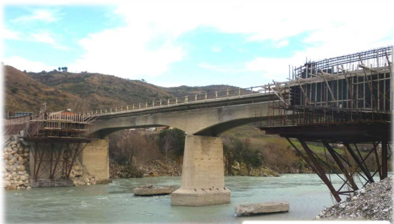
Lot 2 – Bridge under construction at Km 25+185
