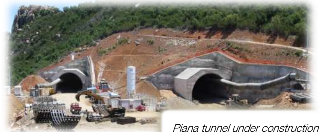
Piana tunnel under construction
