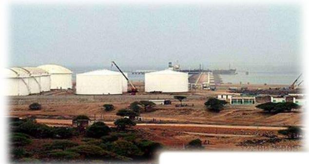
The new oil terminal in operation
