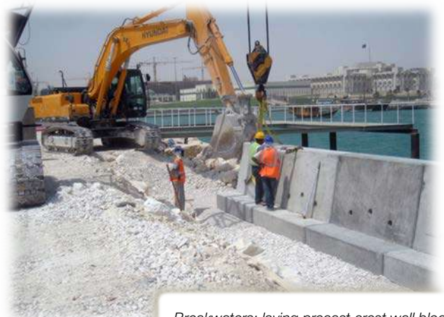
Breakwaters: laying precast crest wall block.
