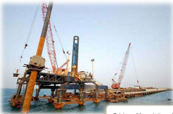
Driving of foundation piles
