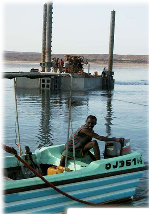
Execution of geotechnical bores at sea
