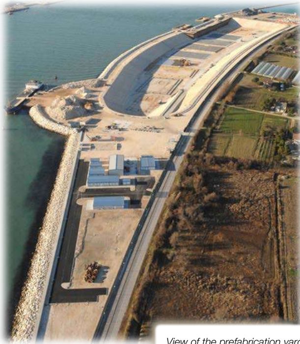
View of the prefabrication yard
