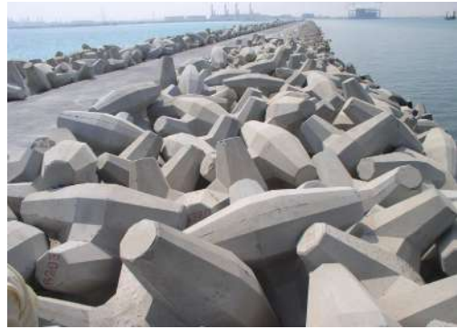
Breakwater – Port of Ras Laffan -Qatar
