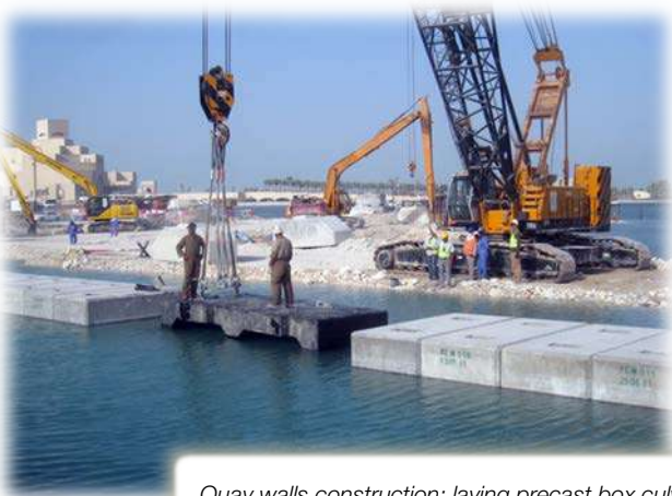
Quay walls construction: laying precast box culvert.
