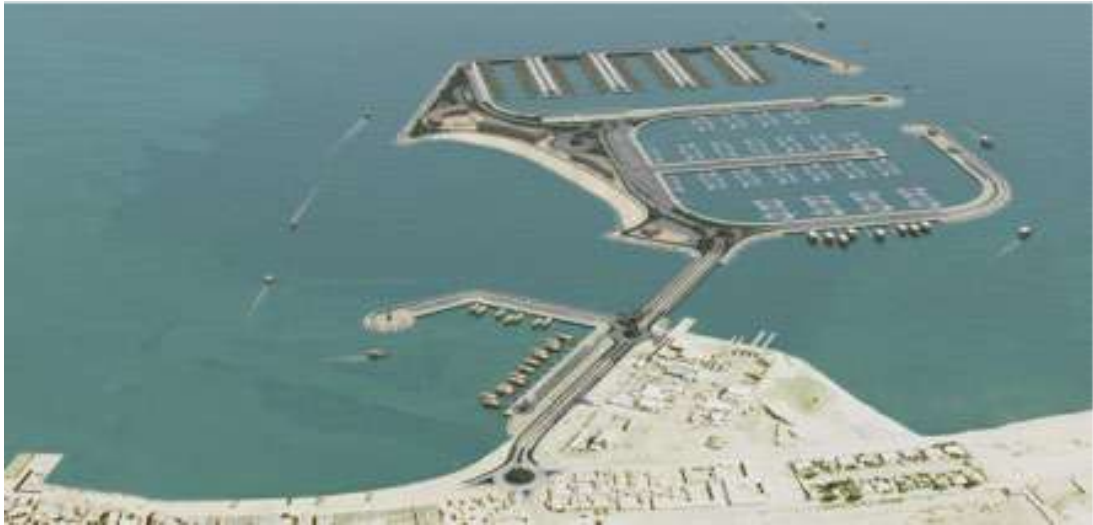
Expansion of Al Wakrah port - Qatar
