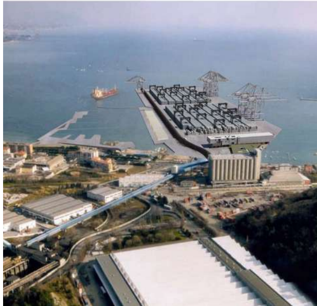
Multipurpose Platform in Vado Ligure– Italy
