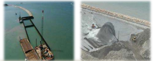
Construction phases of the refugee harbour: cofferdam sheet pile driving and reclamation filling
