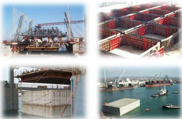
Typical construction, assembly and transportation phases for pre-cast reinforced concrete caisson
