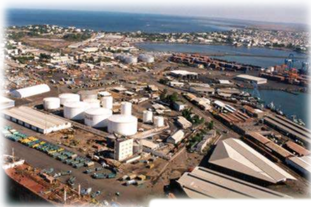
View of the existing oil storage area
