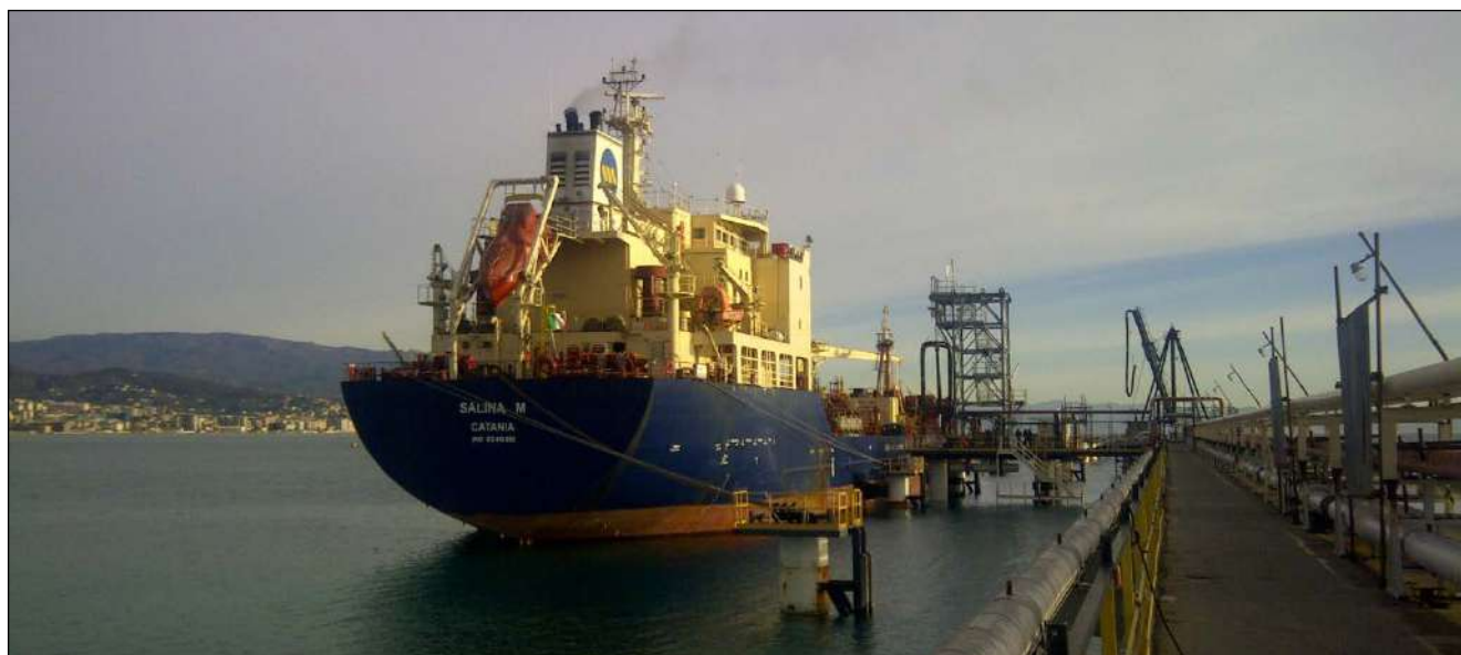
New Exxon berth - View
