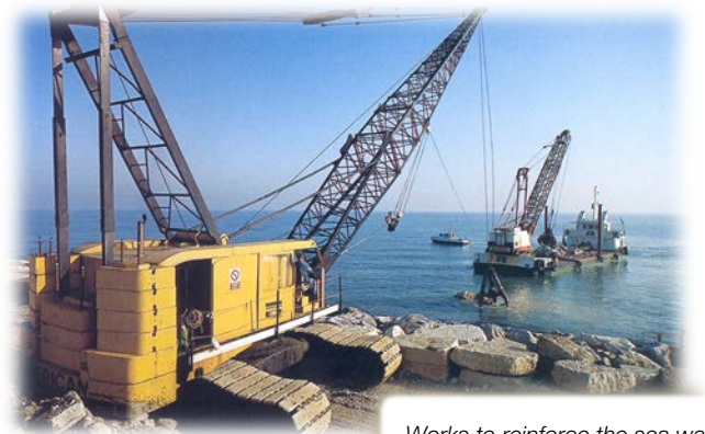
Works to reinforce the sea wall
