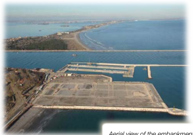
Aerial view of the embankment
