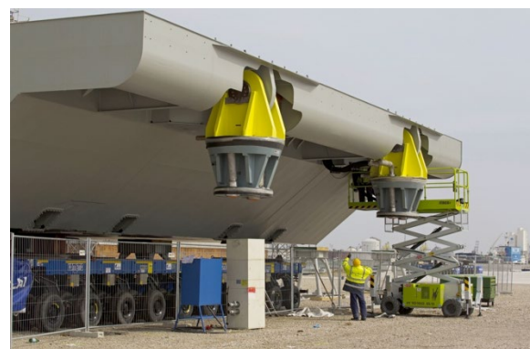
Steel mobile surge barriers
