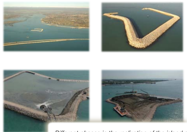
Different phases in the realization of the island core
