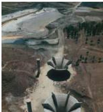
Morning glory spillway Gibbsi Dam
