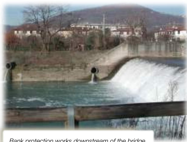
Bank protection works downstream of the bridge
