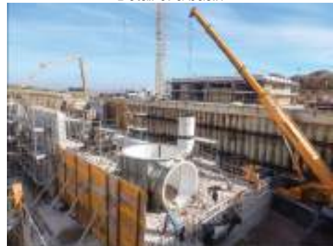
Detail of the main pipe construction
