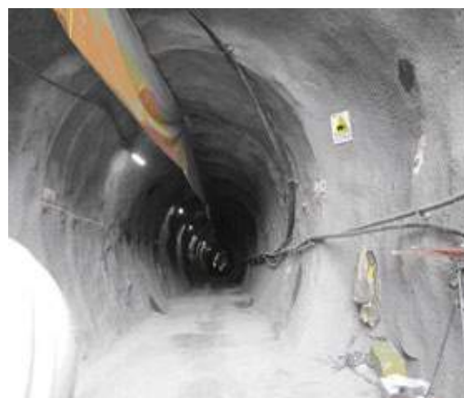
Bottom discharge tunnel of Misicuni Dam
