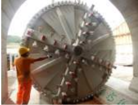
Detail of the TBM
