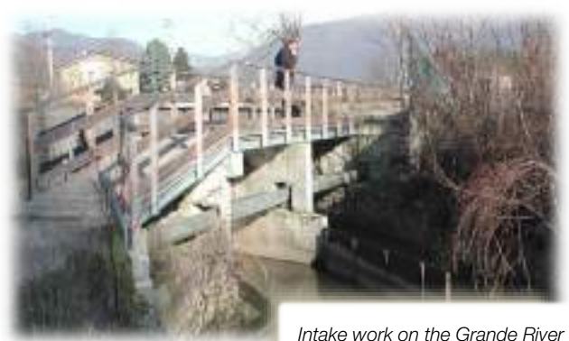
Intake work on the Grande River
