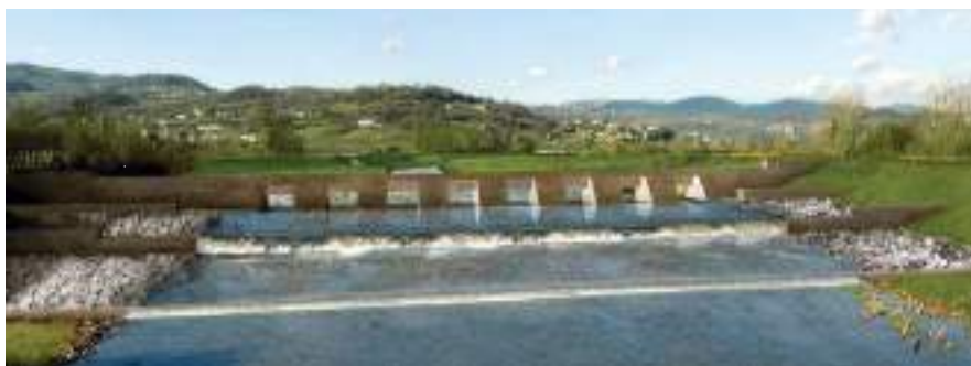
Eight gates connection structure
