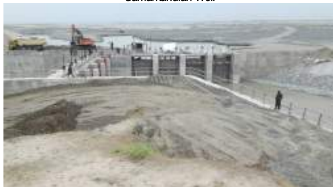
Yetim Tapa Channel Weir
