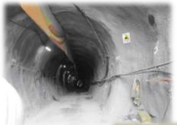
Bottom discharge tunnel
