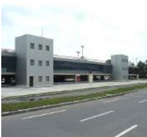
Multi-level car parking of Bucarest Otopeni Airport
