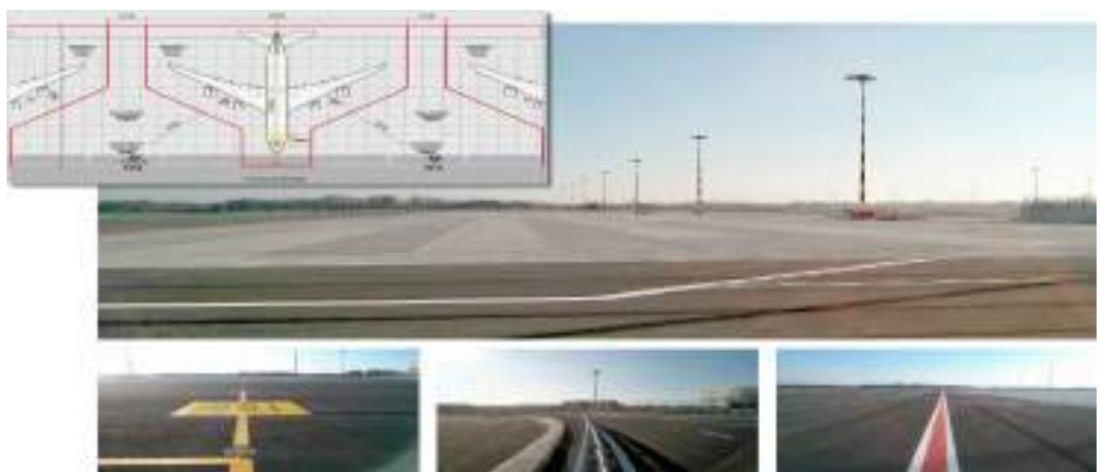
New cargo apron of Milan Malpensa Airport
