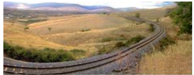
Viaduct "Brancatello" – Current
