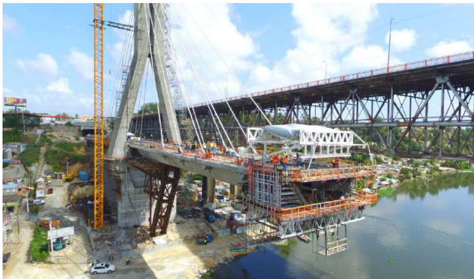
Cable Stayed Bridge on the Light Rail Line, Santo Domingo
